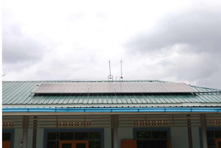
PV Module Capacity (575Wp x 6 Module) Rooftop
